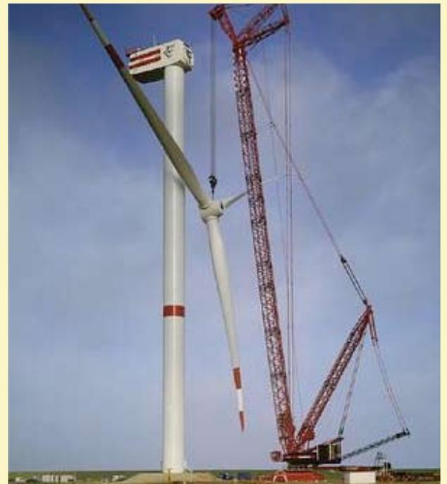
*Liebherr LR. 13500 Crawler Crane erecting Wind Turbine Blades, by the hub*
