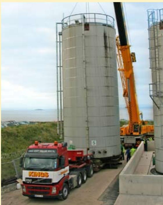
*Kings Heavy Haulage recently moved silos (16.1 m high and 6 m diameter) upright.
